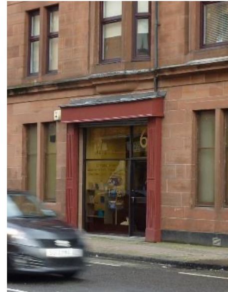
Old tenement building unfit for purpose
